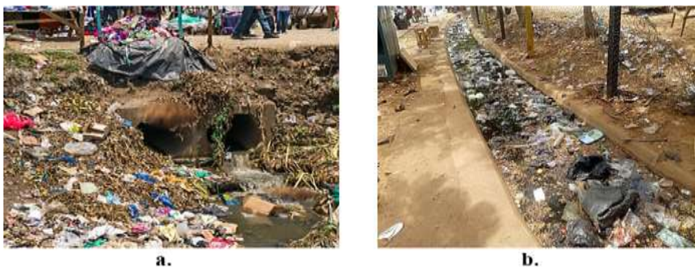
Figure 4: Impacts of plastic wastes on drainage systems
